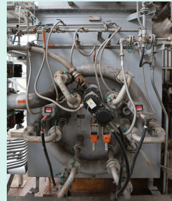
▲ Boiler discharge recovery system
