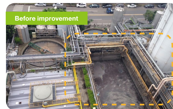
Original #2 aeration pool adopted open air and air diffusion devices for aeration
